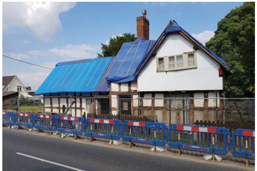
Knoll Cottage, Bircher, Herefordshire, once work began to repair its roof.
