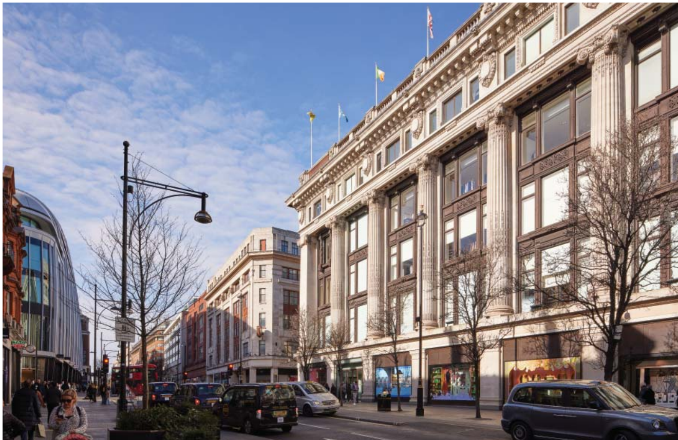
Above and top right: Orchard House, built in 1929, occupies a prominent corner of Oxford Street next to grade II*-listed Selfridge's (Credit: Matthew Andrews for SAVE Britain's Heritage)
