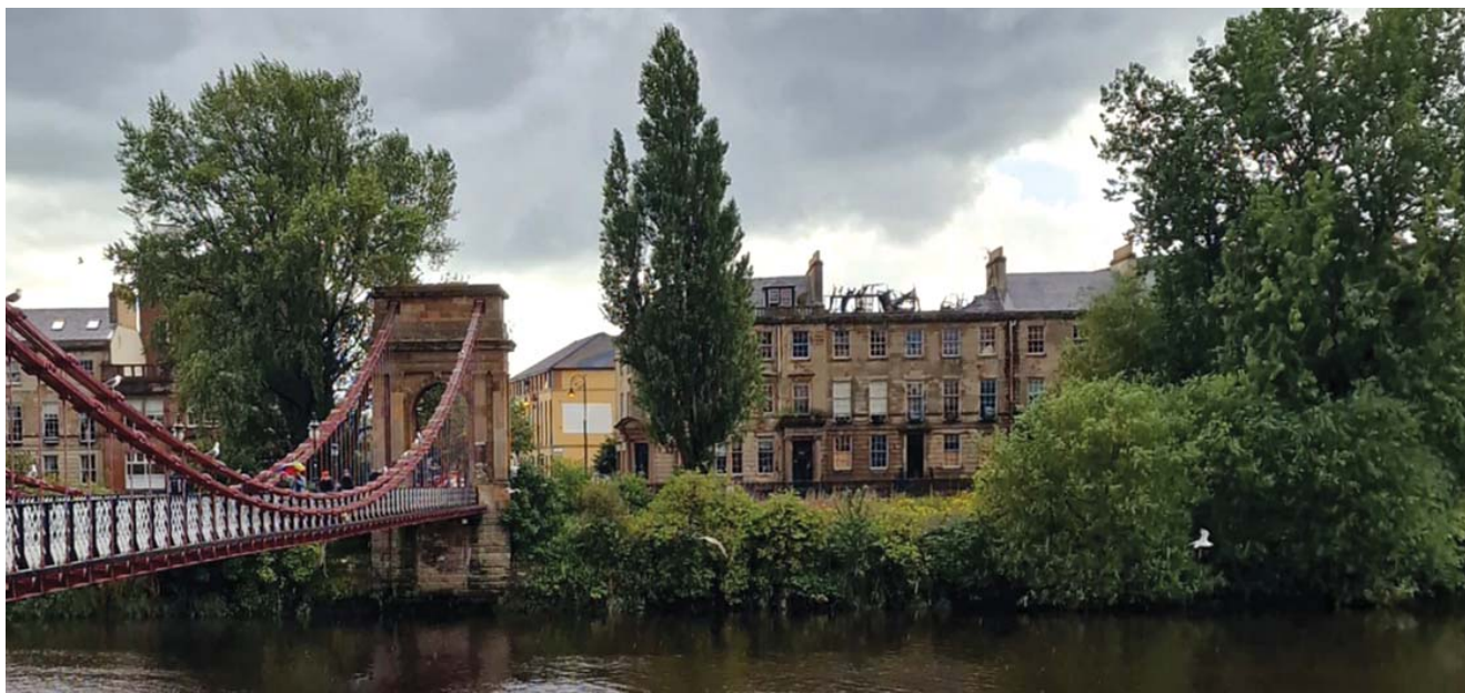
Fire severely damaged the roof of the B-listed former Prince and Princess of Wales Hospice. (Image courtesy of Paul Sweeney)
