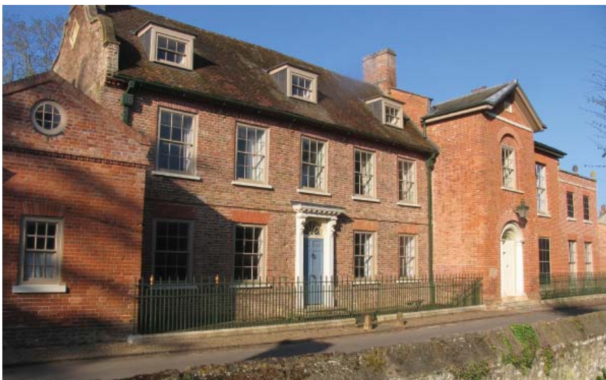
Previous page: Rear elevation and garden post-restoration.
