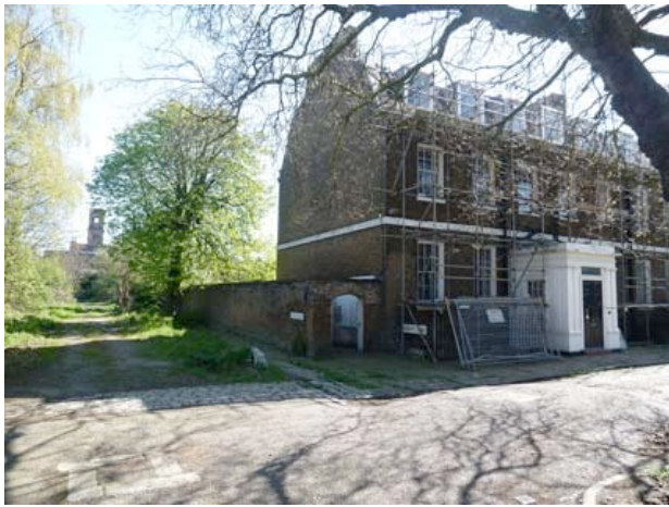
View down Church Road towards the derelict St Paul's Church with Dockyard Terrace on the right. Photo: Rupert Wheeler
