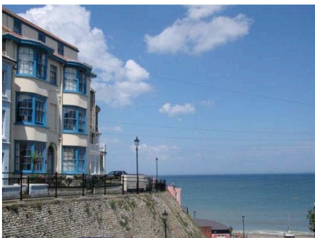
One of Cromer's famous sea views, with The Gangway on the left. The building pictured benefited from a THI grant in 2006.
